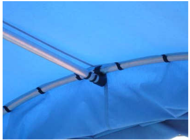
Figure B: Attachment of the canvas to arches using Velcro fasteners
