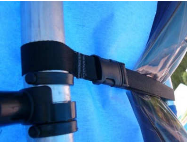
Figure A: Location of the straps of arches on the arch over the coupling (K)
